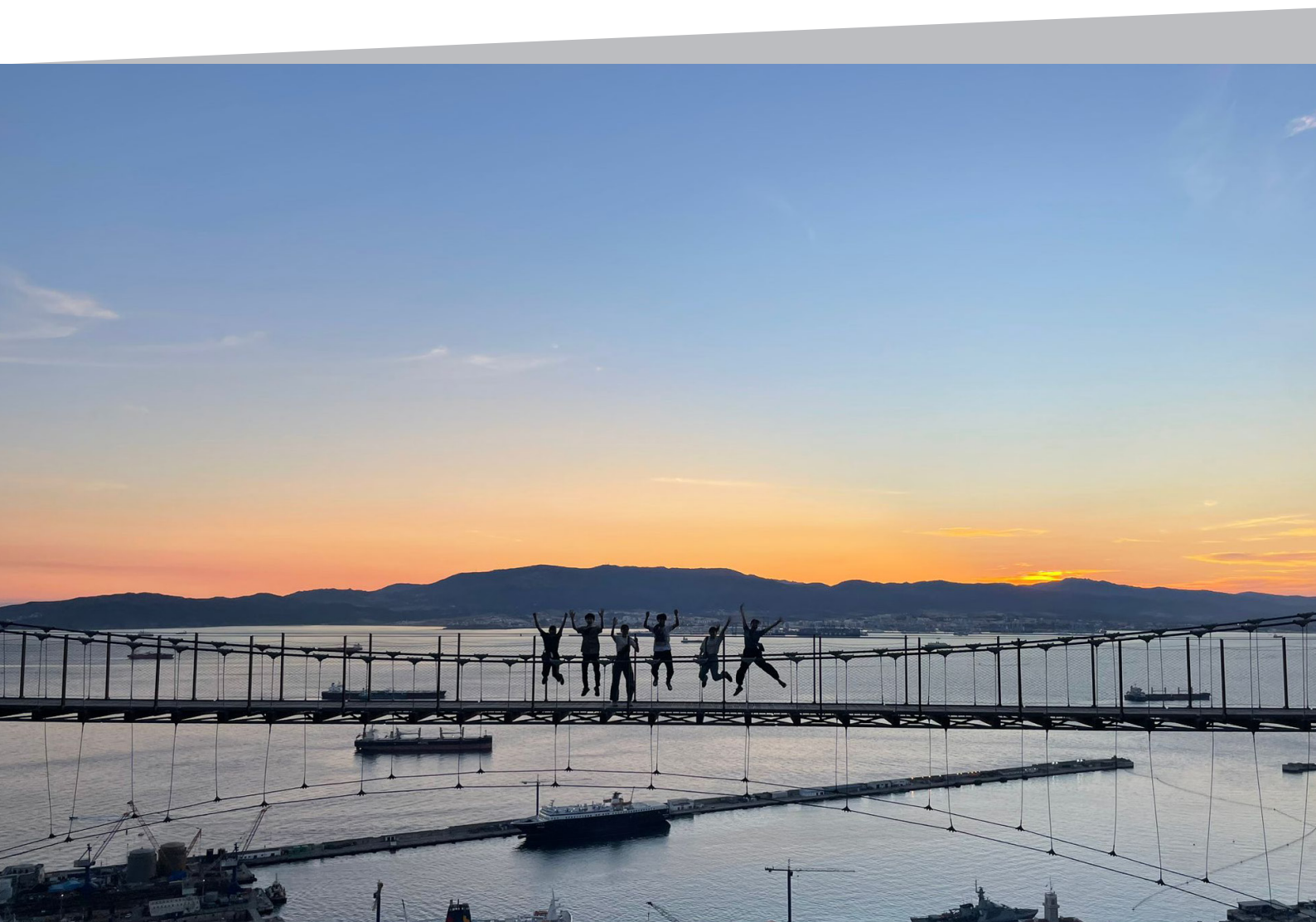
Windsor Suspension Bridge
